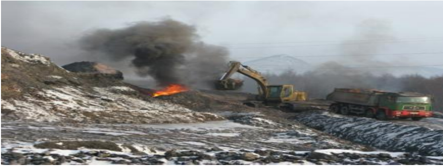
Fig. 4.6. Dismantling of burning coal dump “Wrzosey” [199]
