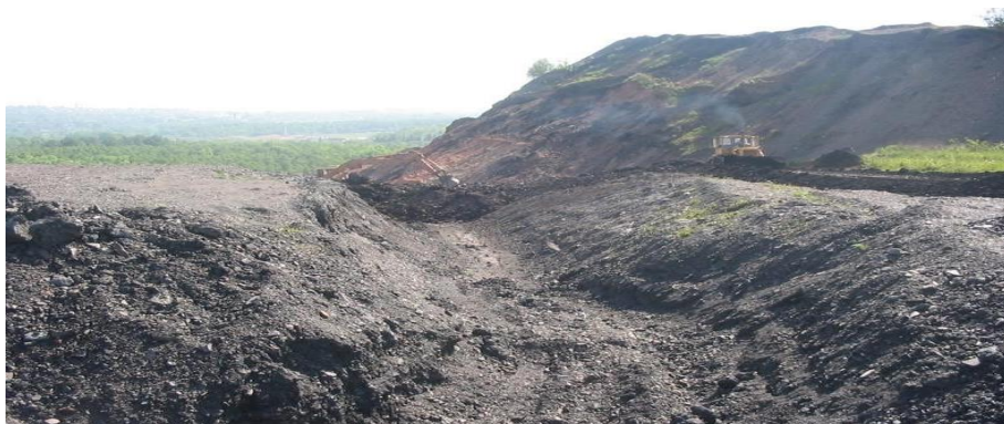
Fig. 4.13. Trench insulating burning part of dump and controlled burning out – Wrzosey “Rydułtowy-Anna” Coal Mine (KWK Rydułtowy-Anna) [source: own]
