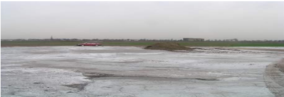
Fig. 4.7. Covering of fire site surface with insulating layer [244]
