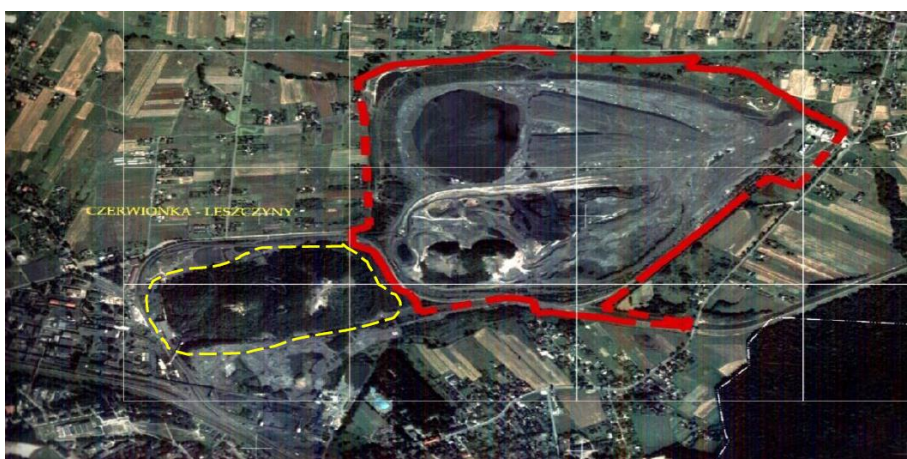
Fig. 5.18. Terrain map of coal dump. Red line marks the area where mining operation is performed. Yellow line marks cones in natural state source: own
