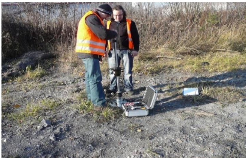
Fig. 5.16. Measurement of soil compaction using Light Weight Deflectometer [source: own]
